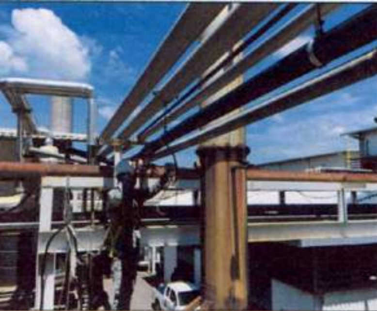
Figure 1: Air quality sampling Boiler Stack No.5 B3
