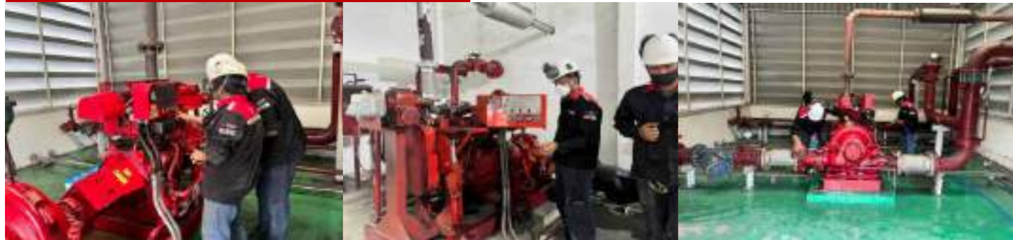
Emergency Equipment and Fire pump Inspection
